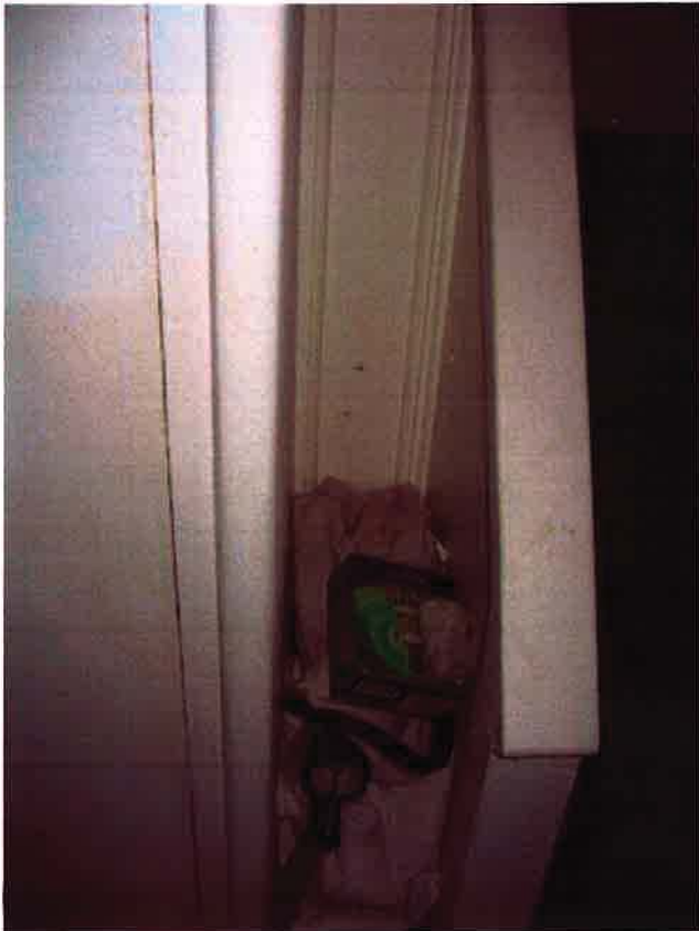
(24) 1st floor stair
